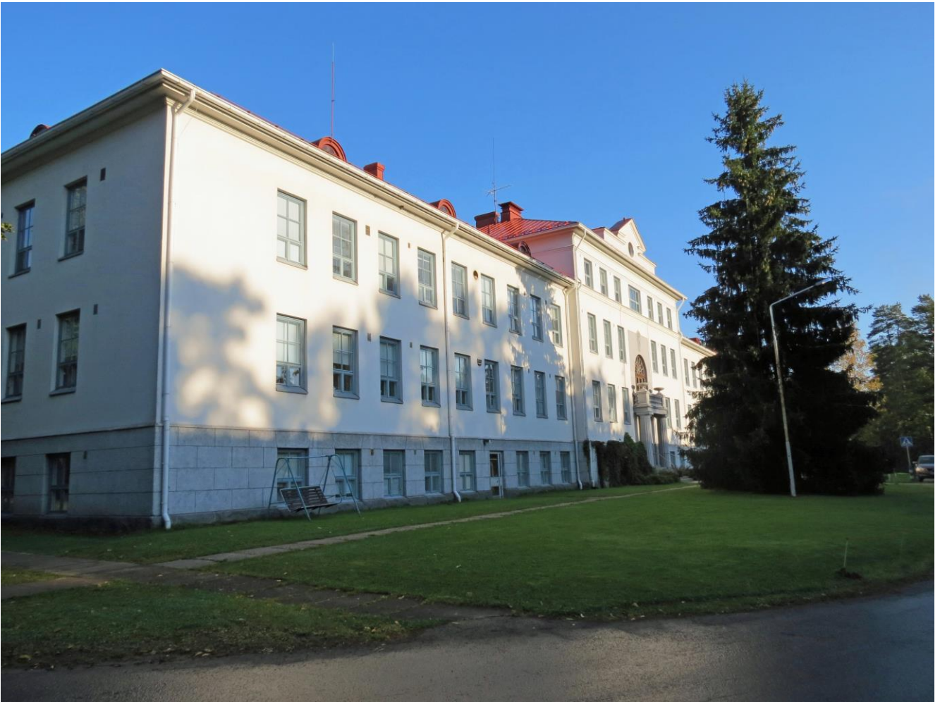
Main building of the Moisio Psychiatric Hospital (Photo by Raimo Kontinen)
